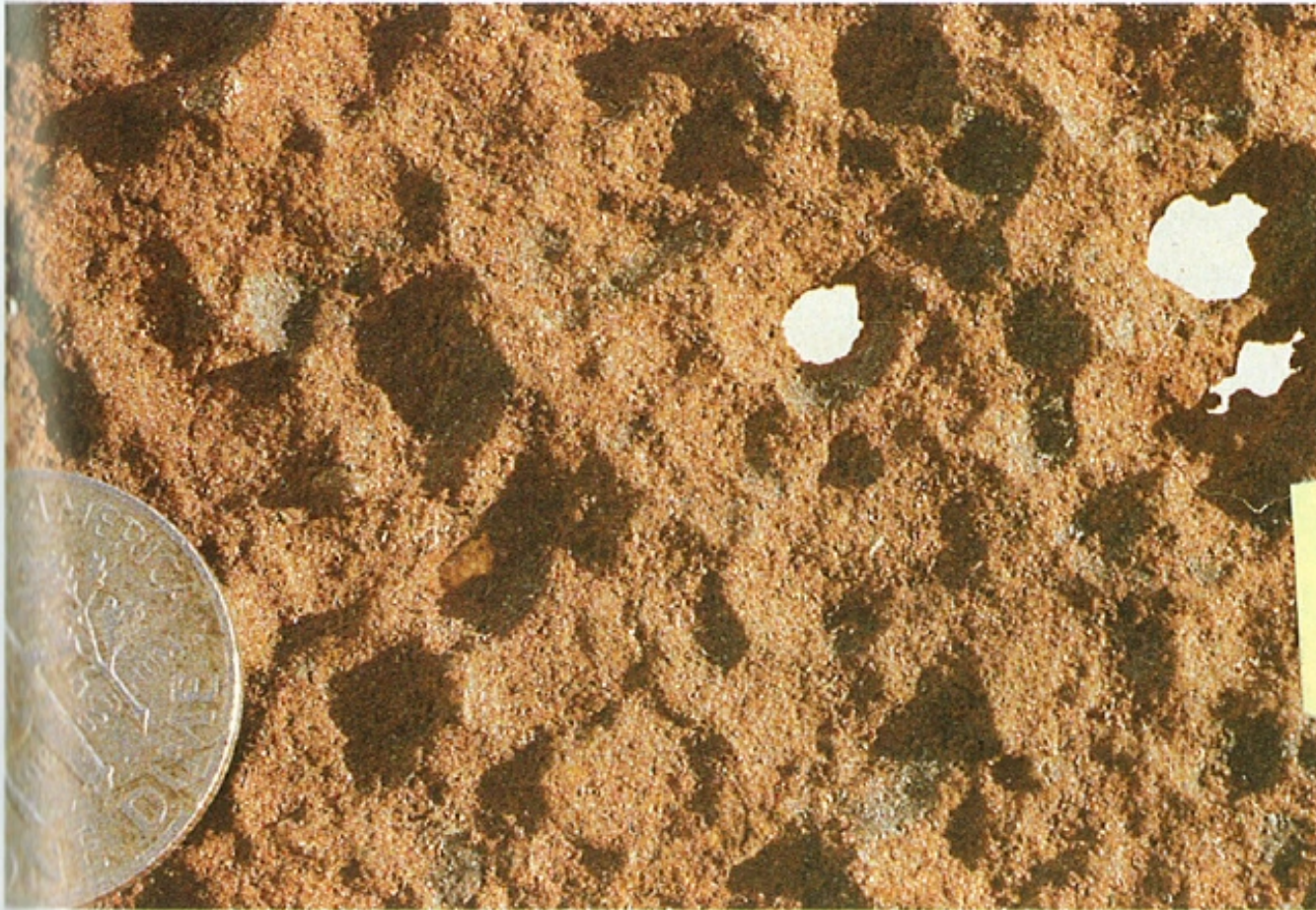
Figure 5.10 Generally corroded steel surface.
