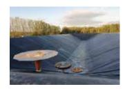
The storage contains 70,000 m<sup>3</sup> water: The length is 180 m, the depth is 14.5 m and the width varies between 52 m and 72 m.
